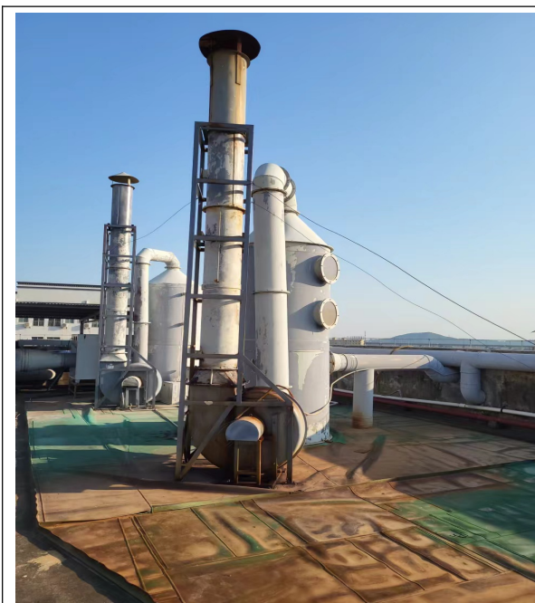
酸雾废气碱喷淋设施
