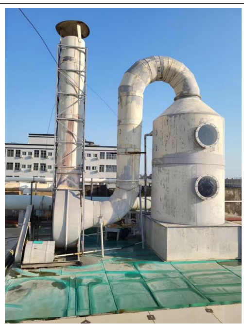
酸雾废气碱喷淋设施
