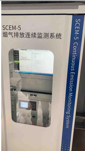
1#-2#石灰窑窑体烟气出口在线监测设施
