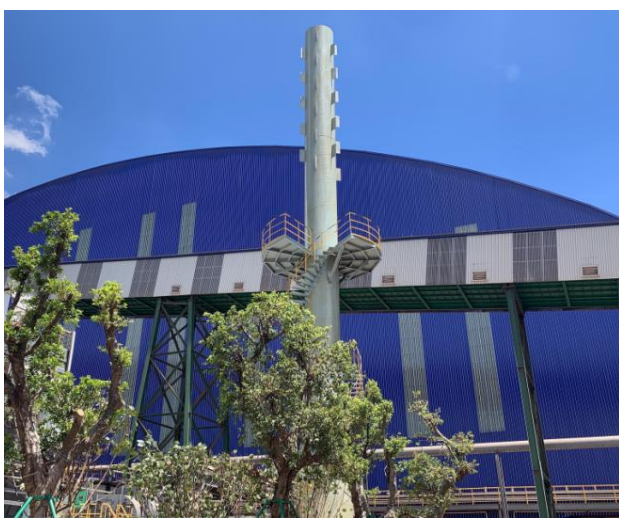
1#-2#石灰窑窑体烟气出口在线监测设施
