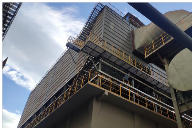
250m 2 烧结机机尾除尘
