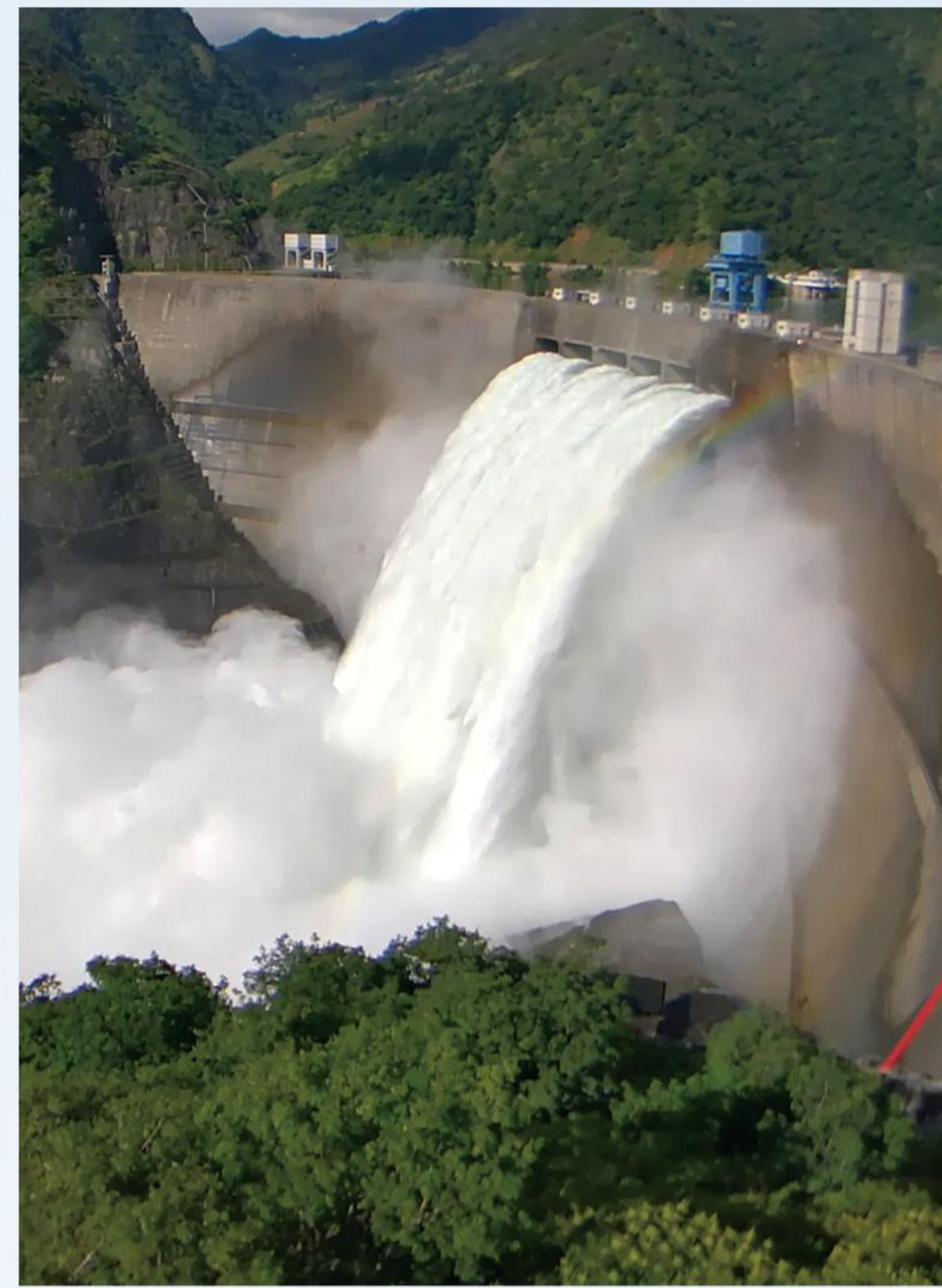
发电 Electric power generation
