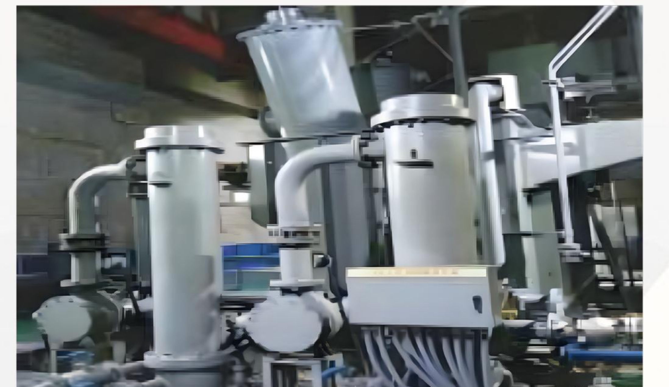
油水冷却器应用于杨家湾水电站 OFAF for Yangjiawan Hydropower Station
