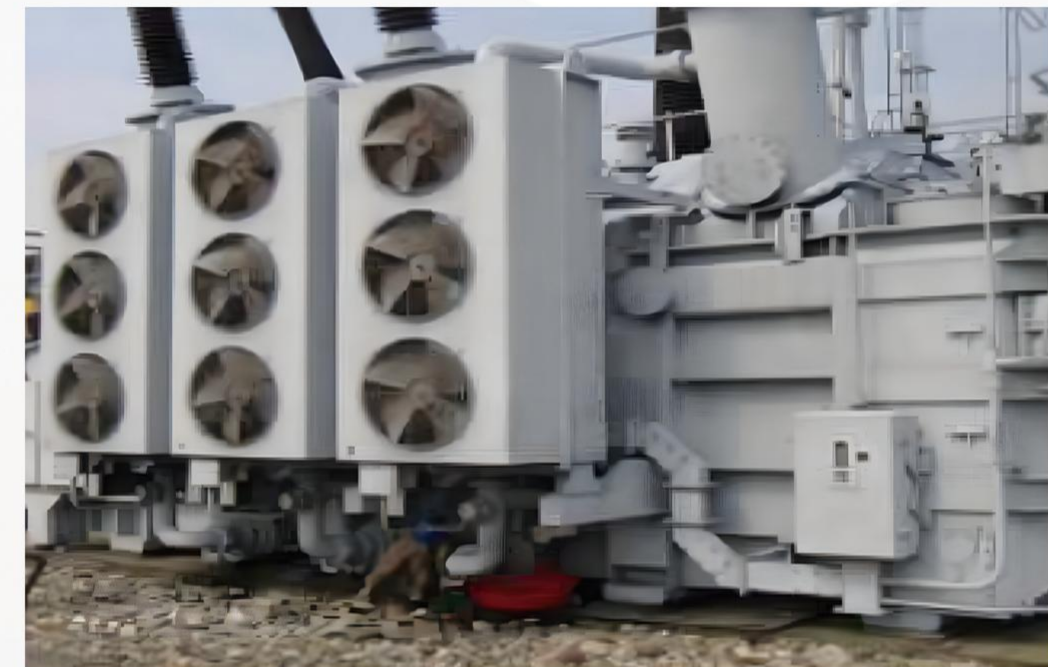
变压器油泵于 2006 年开始应用在长江三峡主变压器冷却系统 Transformer oil pump was applied in the cooling system of the main transformer of the Three Gorges Project in 2006
