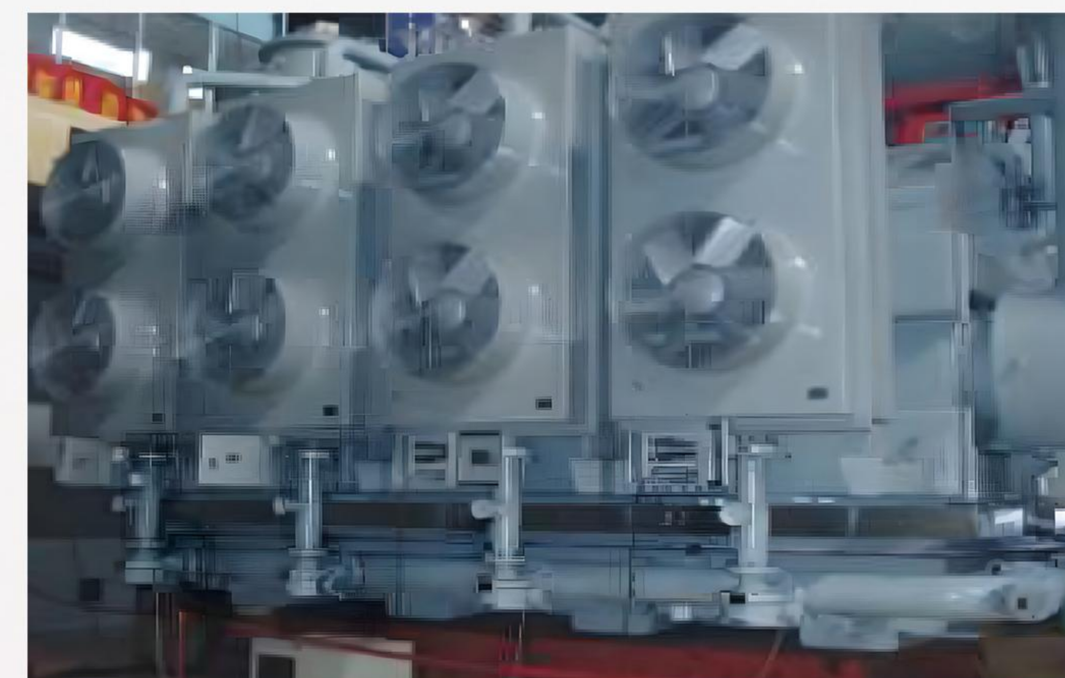
变压器油泵及油流继电器、蝶阀应用于泰山核电站第一座 30 万千瓦压力堆核电站 Transformer oil pump, oil flow relay and butterfly valve are applied to the first 300000kW pressure reactor nuclear power plant in Qinshan Nuclear Power Station
