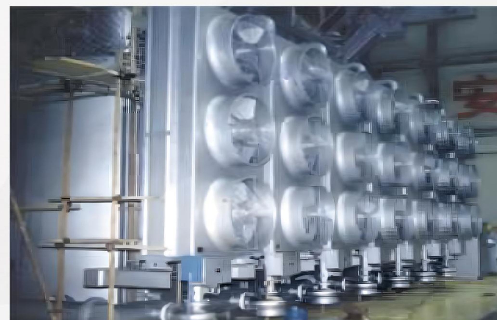
油泵及油流继电器、蝶阀应用于澳大利亚塔隆电厂采用的常州东芝 500 千伏安变压器中 oil pump, oil flow relay and butterfly valve matched with Changzhou Toshiba 500kVA transformer were used in Talon Power Plant, Australia
