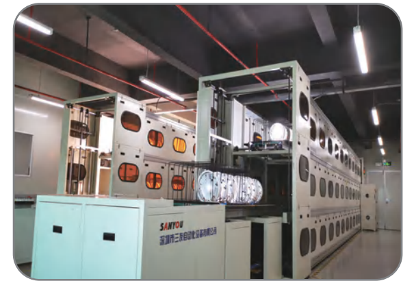
Automatic Aging Line
