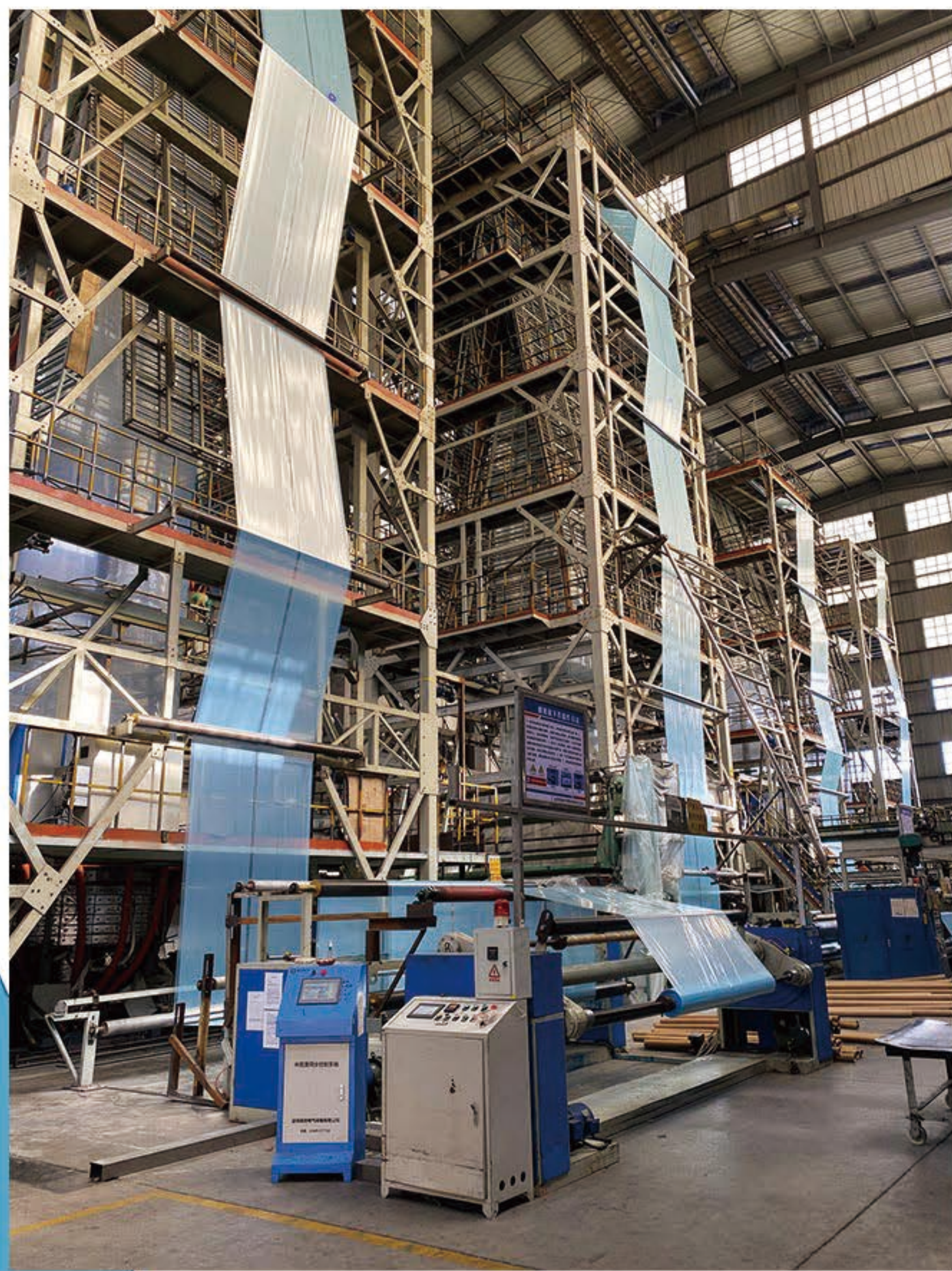
棚膜设备概览 Overview of Shed Film Equipment
