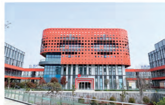
Factory in Jining, Shandong, 60,000m 2
