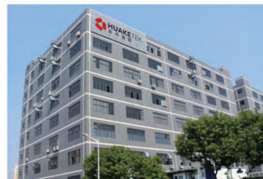
Factory in Shenzhen, Guangdong, 25,000m 2
