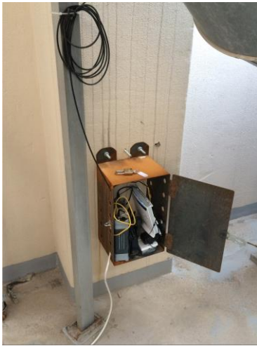
CORS station located nearby the construction site
