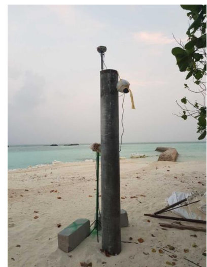
Fig. 4: .Fixing the base on the first pile with known coordinate.
